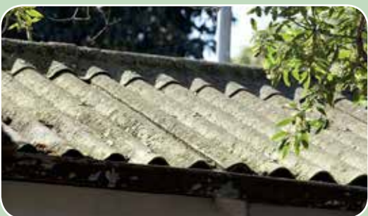
Asbestos cement corrugated roofing
