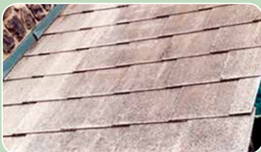
Asbestos cement shingles
