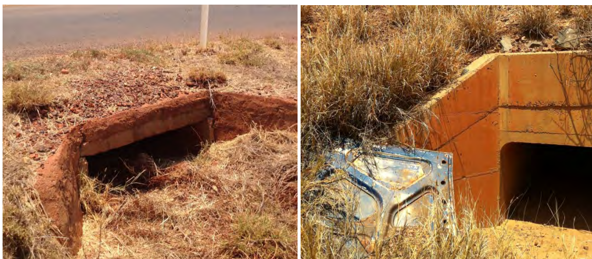
Plate 2: Typical obstructions observed at some culverts
