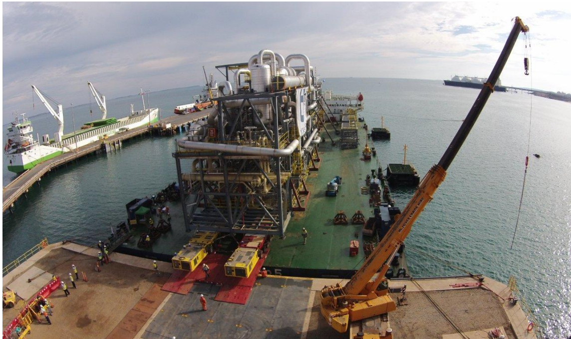
Figure 19: Giant RORO cargo discharged at the FDTs berth.
