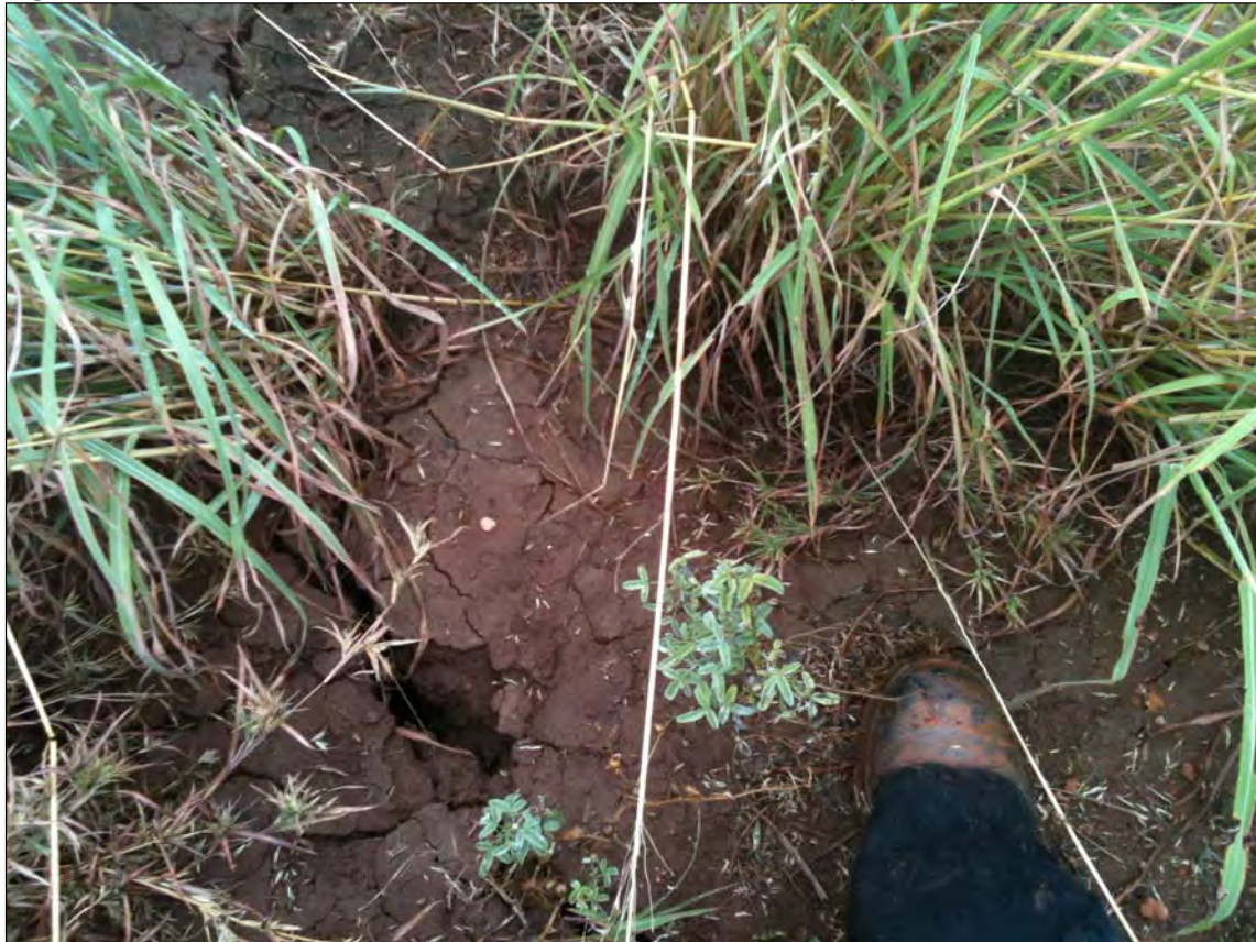
Figure 1: Cracks and 'crab holes' observed in the south-eastern part of the site
