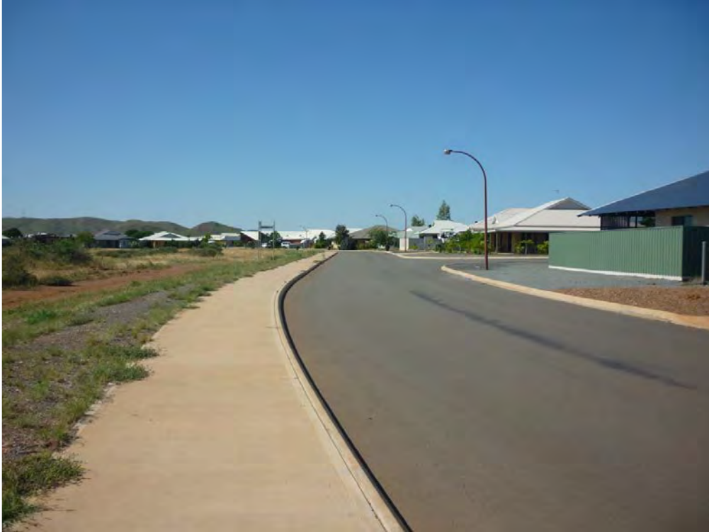
Figure 3 Bowerbird Drive to the south of the site
