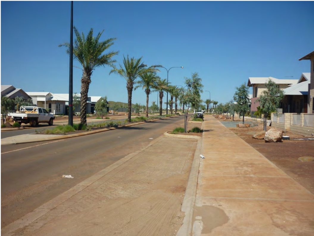
Figure 20 Example of on-street parking provisions
