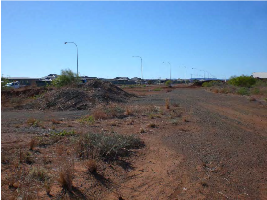
Plate 3: View north adjacent to topsoil (2010).
