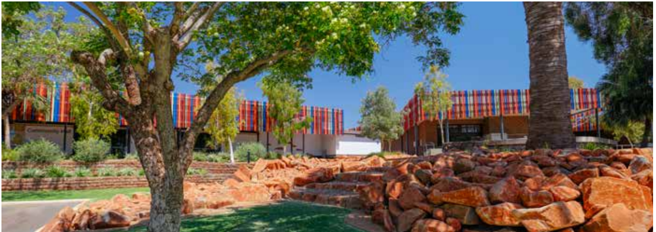
Dampier Community Hub
