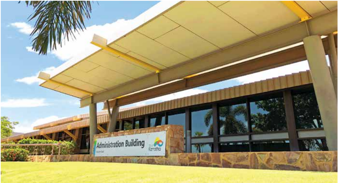
City of Karratha Administration Centre
