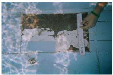
1.15M EXPANSION JOINT - FAILED SEALANT
