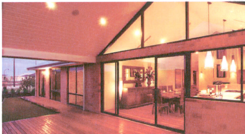
Example of generously sized covered outdoor living area directly accessed from indoor living spaces. Note timber floor finish, timber absorbs less heat than paving, keeping area cooler. See 7.1.1. (Image Rural Building Co.)
