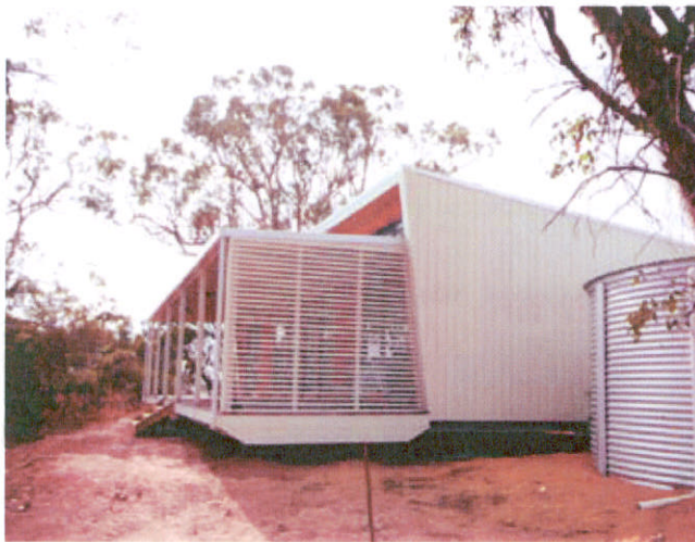
Example of high quality transportable home. Note breeze wall, high capacity rain water tank and light coloured roofing/cladding material. Please also note that eave width does not comply with eave width requirements. (image, Nordic Homes), See 7.6.2, 7.9.3, & 7.1.6/7.1.7
