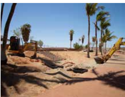
Commencement of the Dampier foreshore redevelopment
