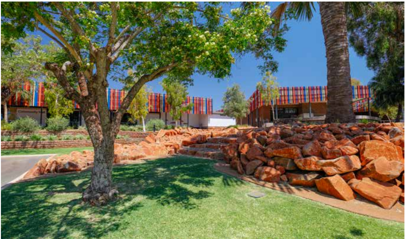
Dampier Community Hub
