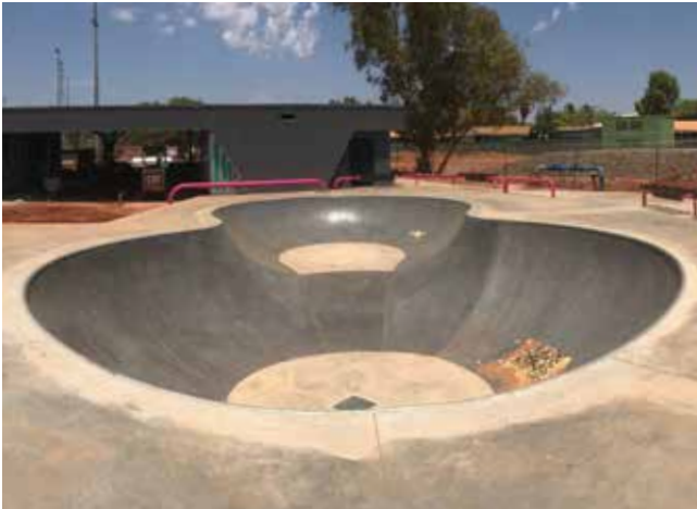
Wickham Community Hub Skate Park under construction
