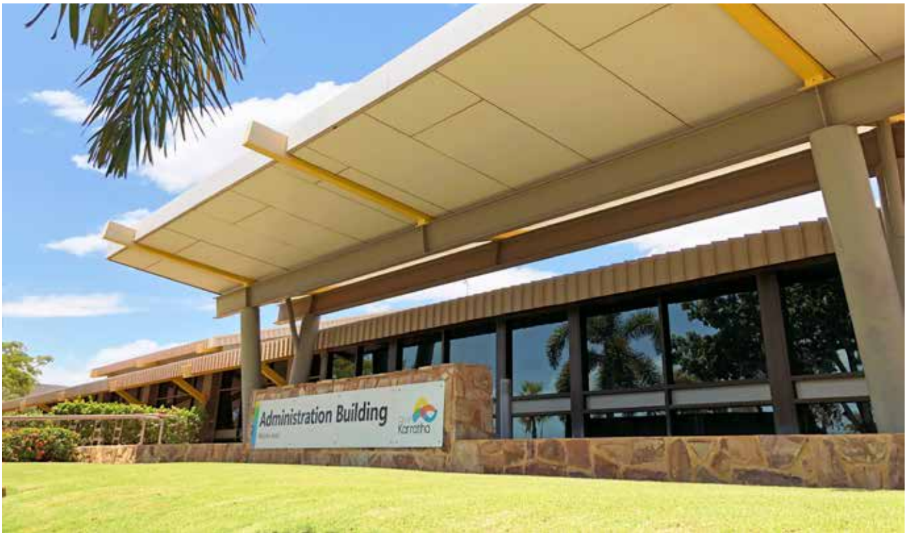
City of Karratha Administration Centre
