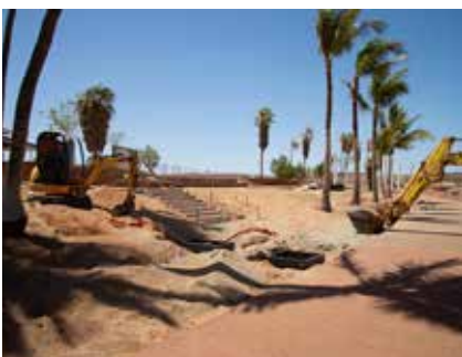
Commencement of the Dampier foreshore redevelopment
