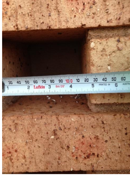
Double Niche opening 100mm (H) x 255mm (W)
