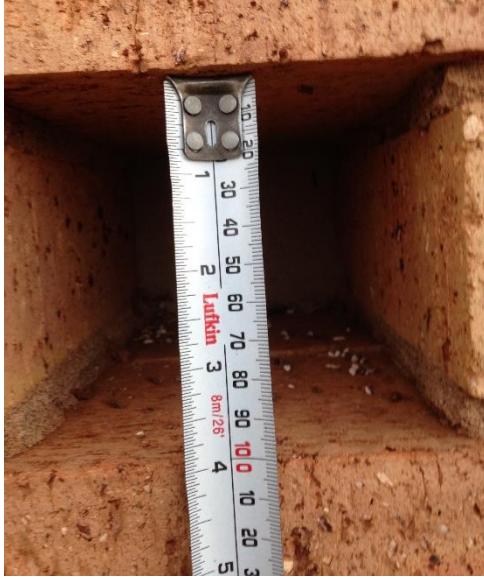
Double Niche opening 100mm (H) x 255mm (W)
