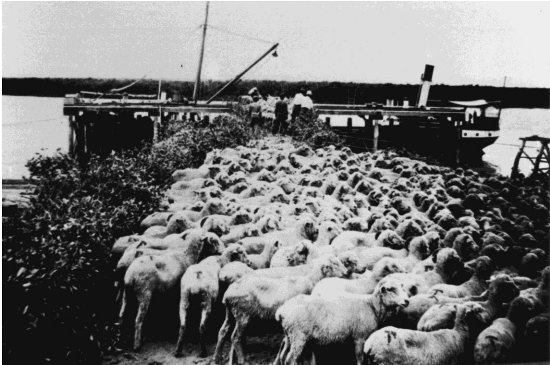
Sheep being loaded at Balla Balla jetty (Courtesy Shire of Roebourne Local History Collection, 2005.126)
